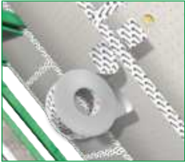
Bonding overlaps and injection holes
