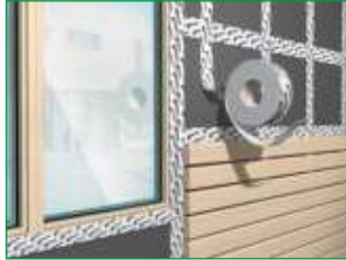
Sealing exterior roof and facade sheeting
